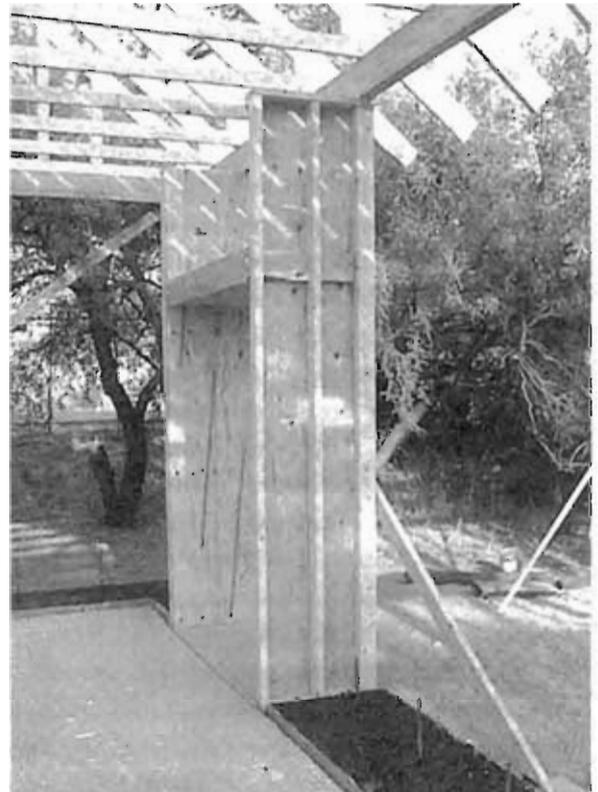
Figure 7-9. Modified post-and-beam, in-fill wall structure. Illustration from *The Straw Bale House* by Athena Swentzell Steen, Bill Steen, and David Brainbridge with David Eisenberg (Chelsea Green Publishing Company, 1994).
